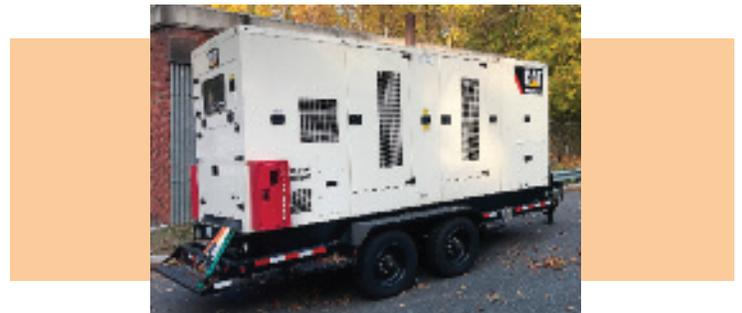
The Authority recently purchased a new portable generator to provide emergency redundancy back-up power at multiple locations. Manual transfer switches and plugs have been installed at remote well sites, so the portable unit can be deployed as needed and quickly connected to support the Authority's distribution system at short notice.
