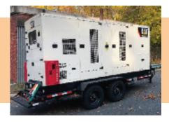
The Authority recently purchased a new portable generator to provide emergency redundancy back-up power at multiple locations. Manual transfer switches and plugs have been installed at remote well sites, so the portable unit can be deployed as needed and quickly connected to support the Authority's distribution system at short notice.
